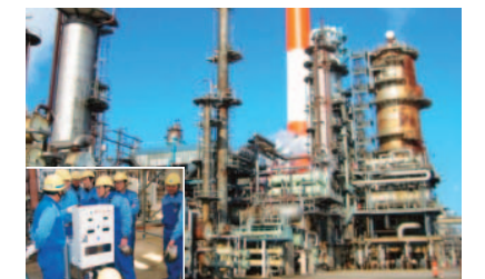
Refinery turbine lubricating oil (SRC-814-15V; explosion proof)
